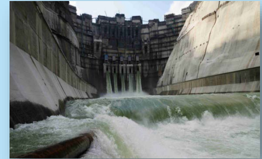
Jinping I, 305m high
