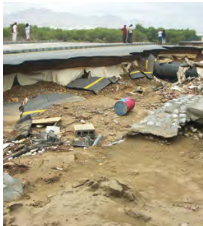
Damages in Muscat after the passage of Cyclone Gonu, Oman, 2007. Source: Wikimedia Commons.
