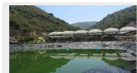
Rainwater from greenhouses is stored in ponds to be used for irrigation in other greenhouses
