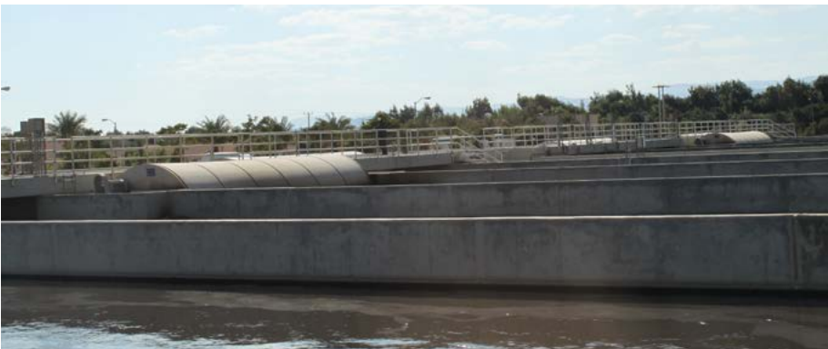
Photo Credit: Jordan Wastewater Treatment Plant, ACWUA, 2016
