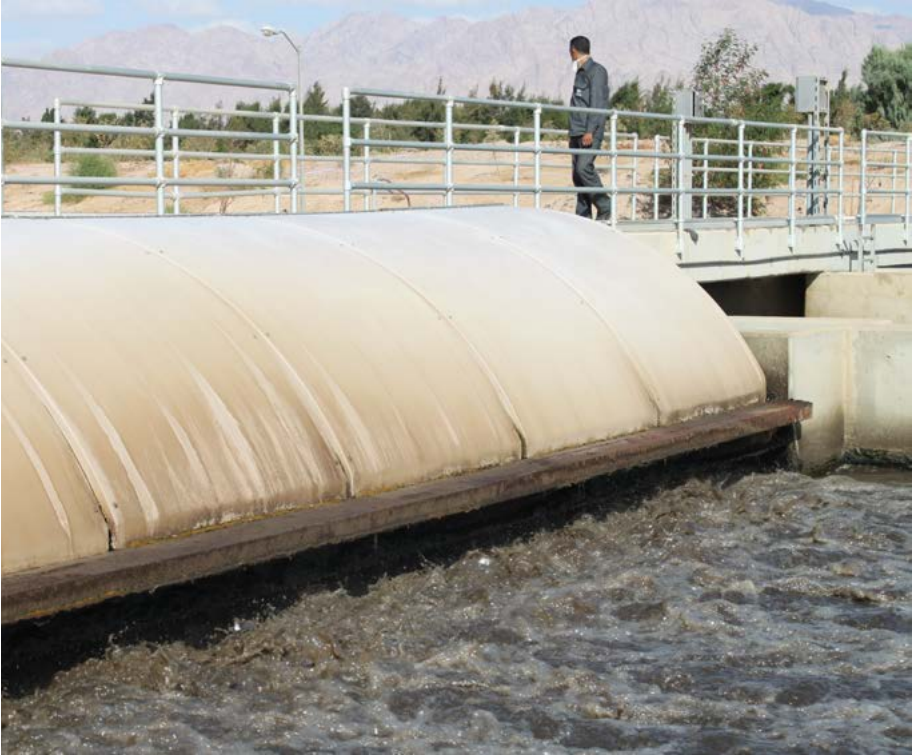
Photo Credit: Jordan Wastewater Treatment Plant, ACWUA, 2016
