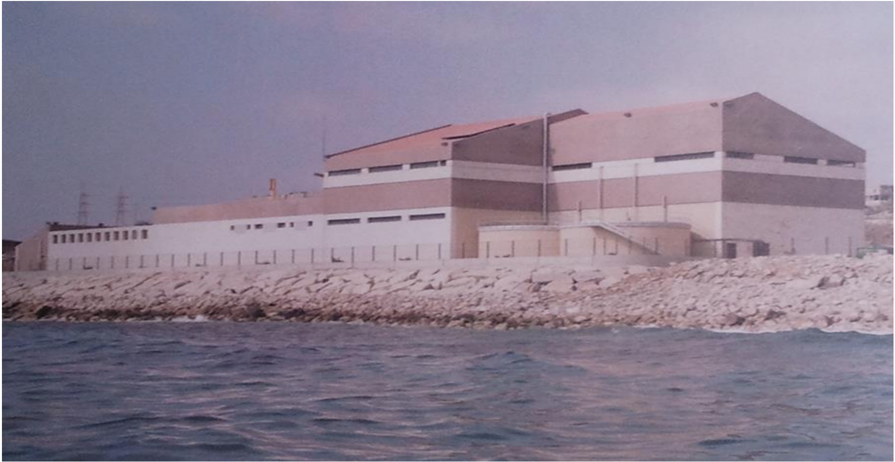
Jieh Waste Water Treatment Plant
