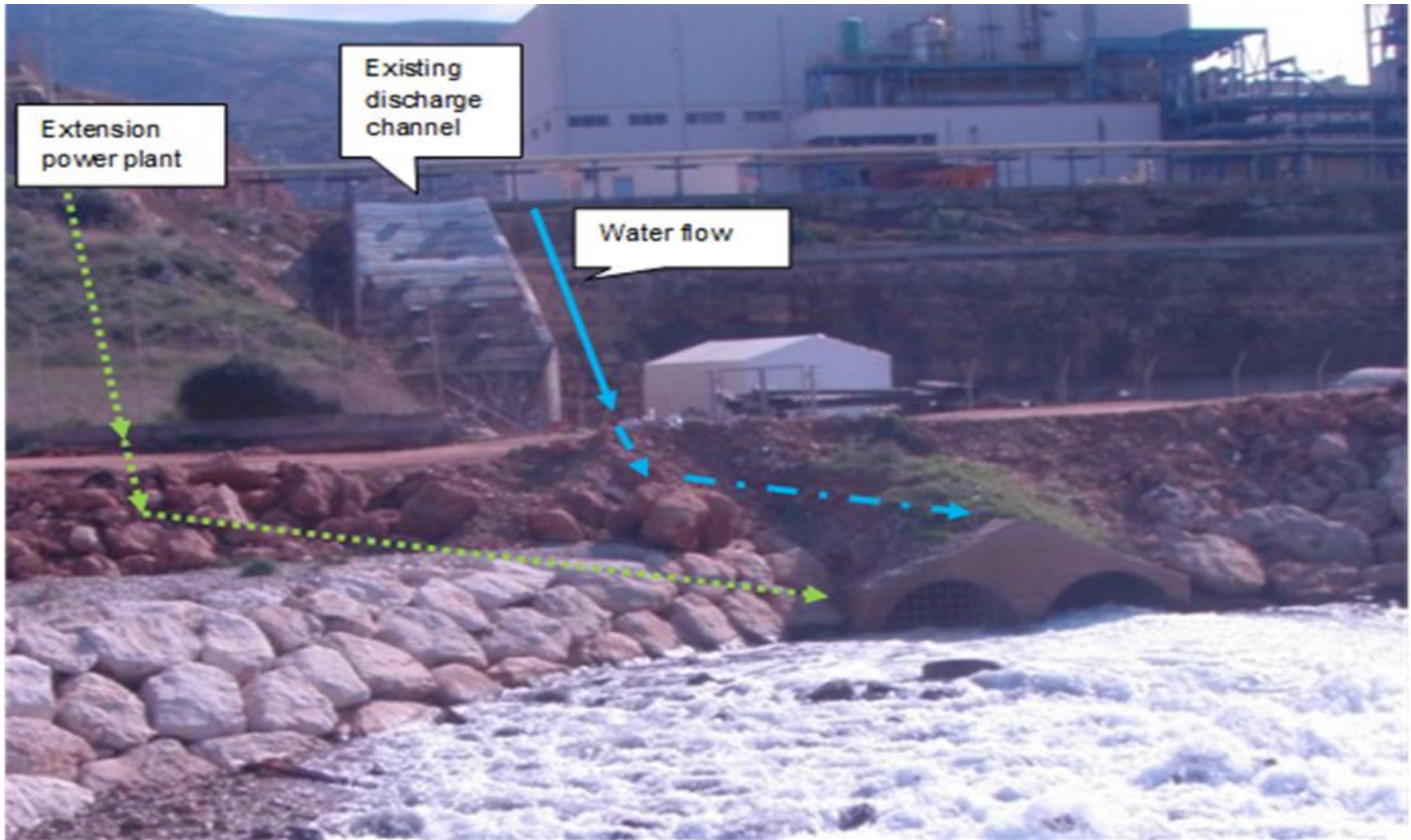
Deir Ammar Combined Cycle Power Plant Outfall Channel
