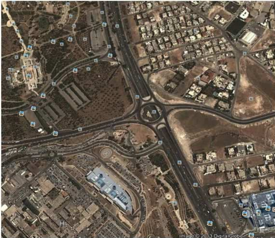
Figure 20: Land use features dictate value of the Runoff coefficient for storm sewer design, AlMadeena Tunnel, Amman Jordan
