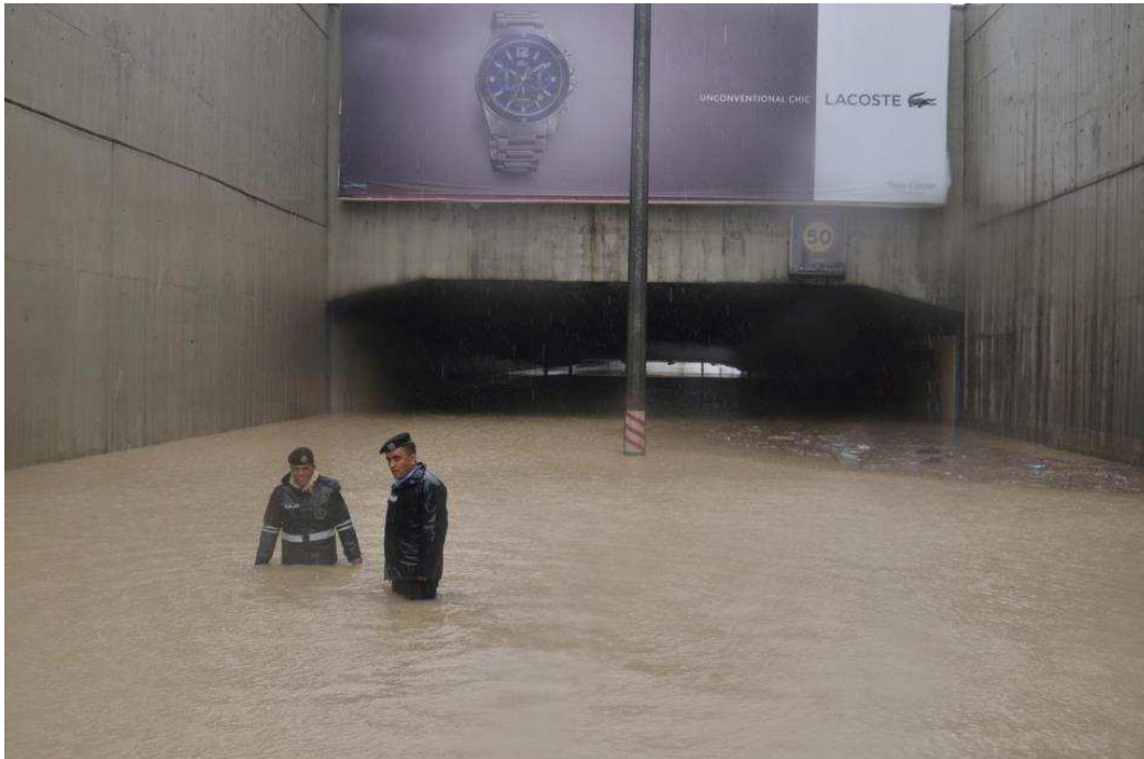
Figure 19 : Street tunnel flooded with storm water in West Amman, winter 2014
