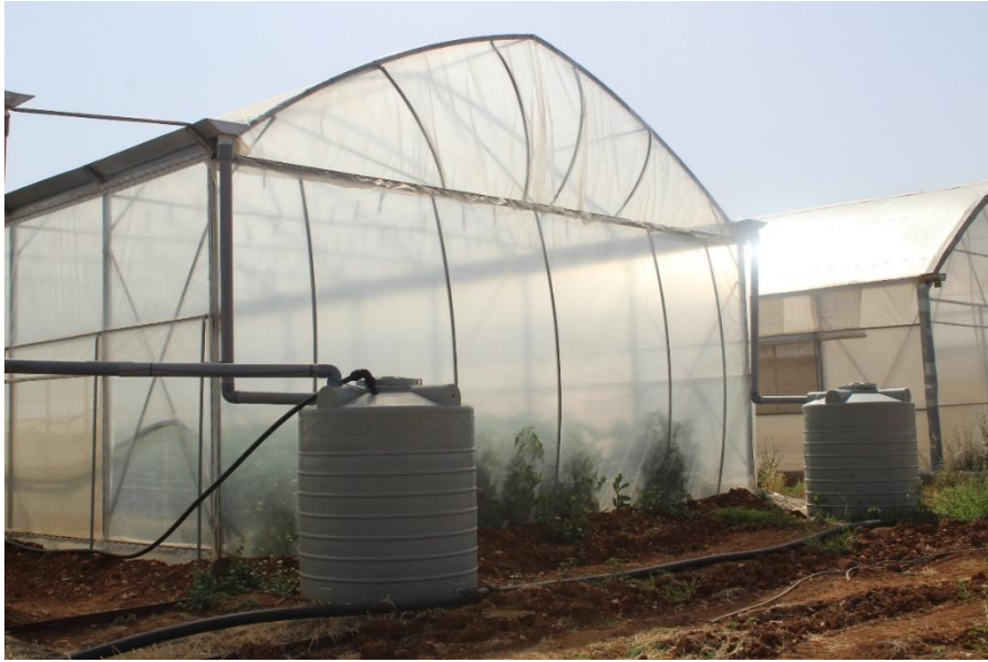
Gutter based rainwater harvesting system
