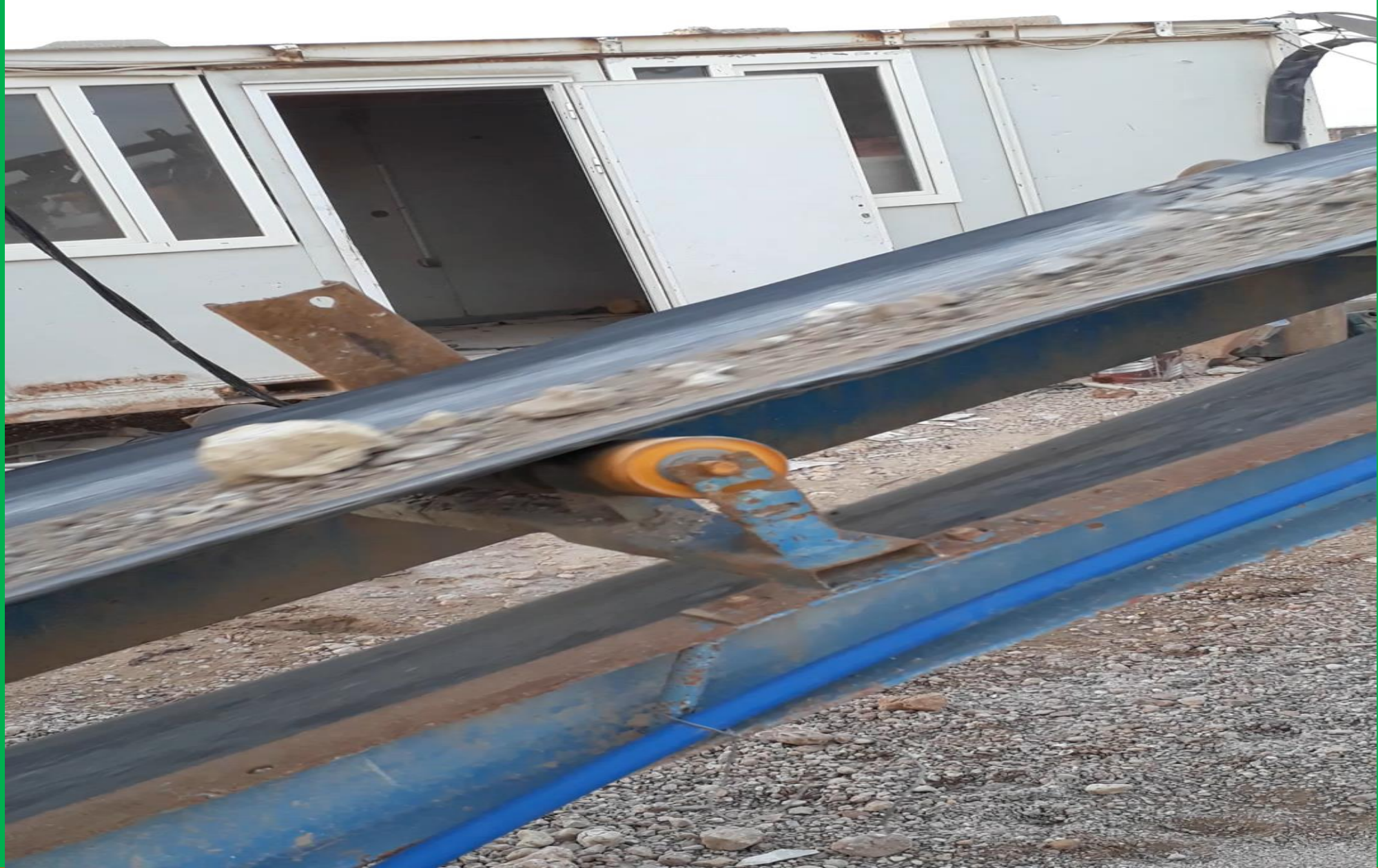
Crushing of debris
