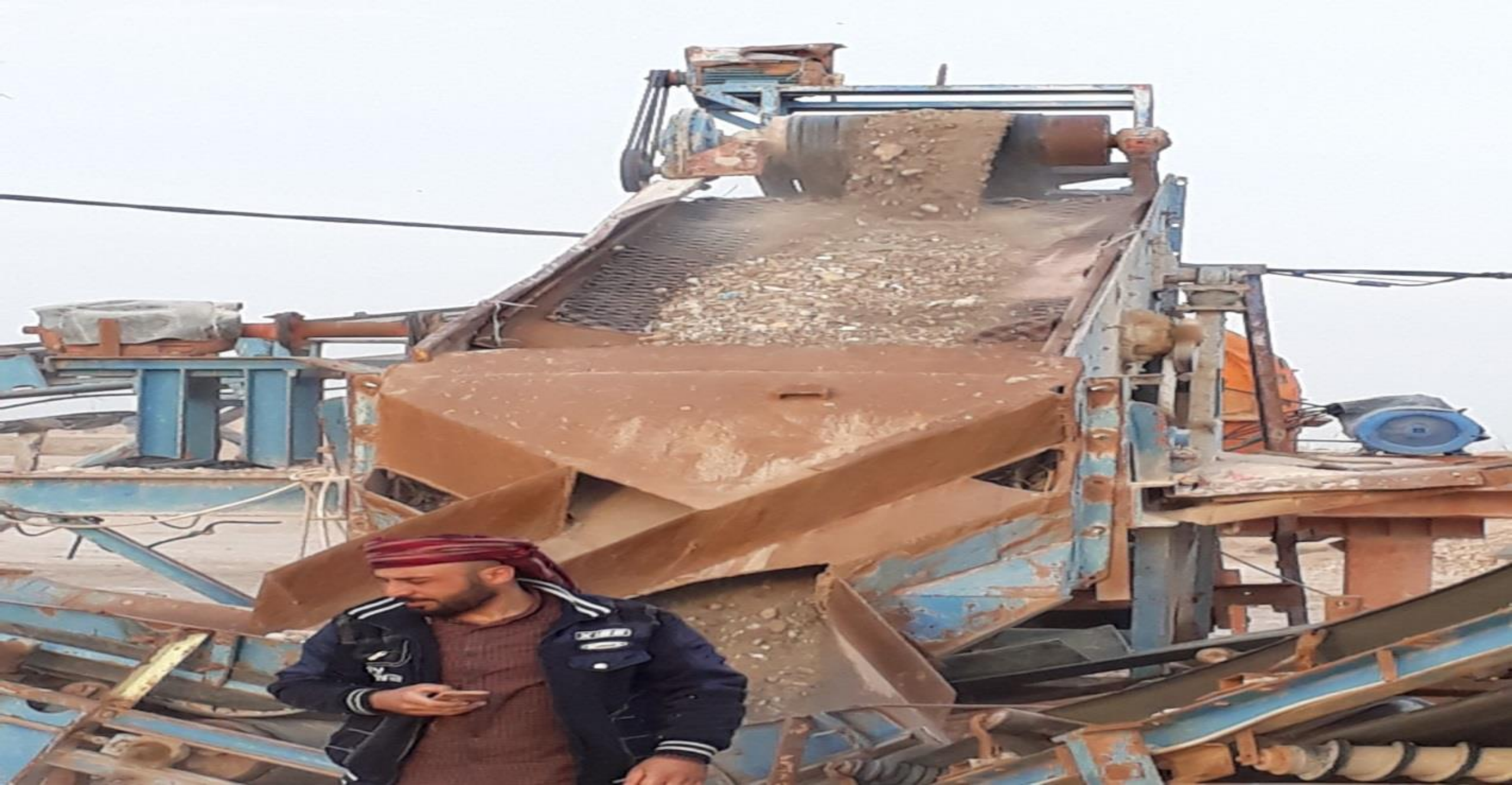
Photo 9. show the demolition waste subbase on the sieve after crashing
