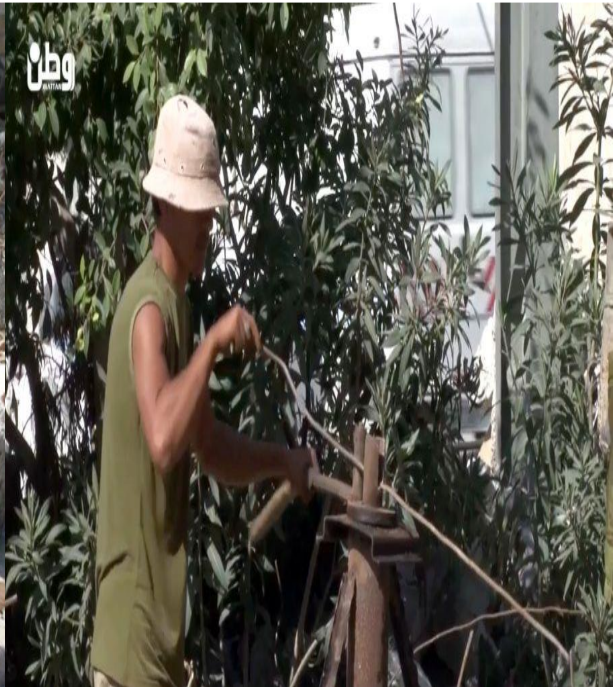
3-Re-adjustment of steel bars
