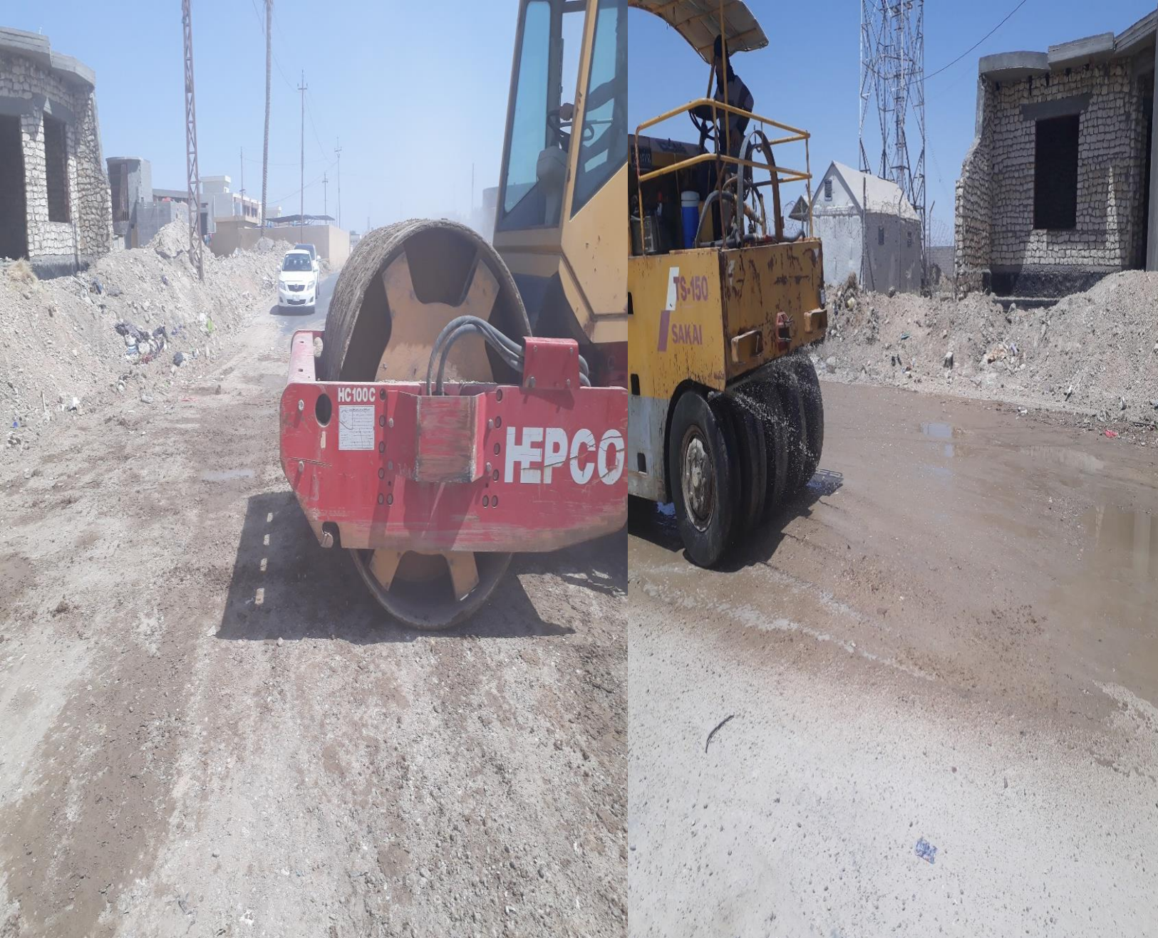
Photo 13,14,15 shows the sprinkle with water , compaction and test the samples
