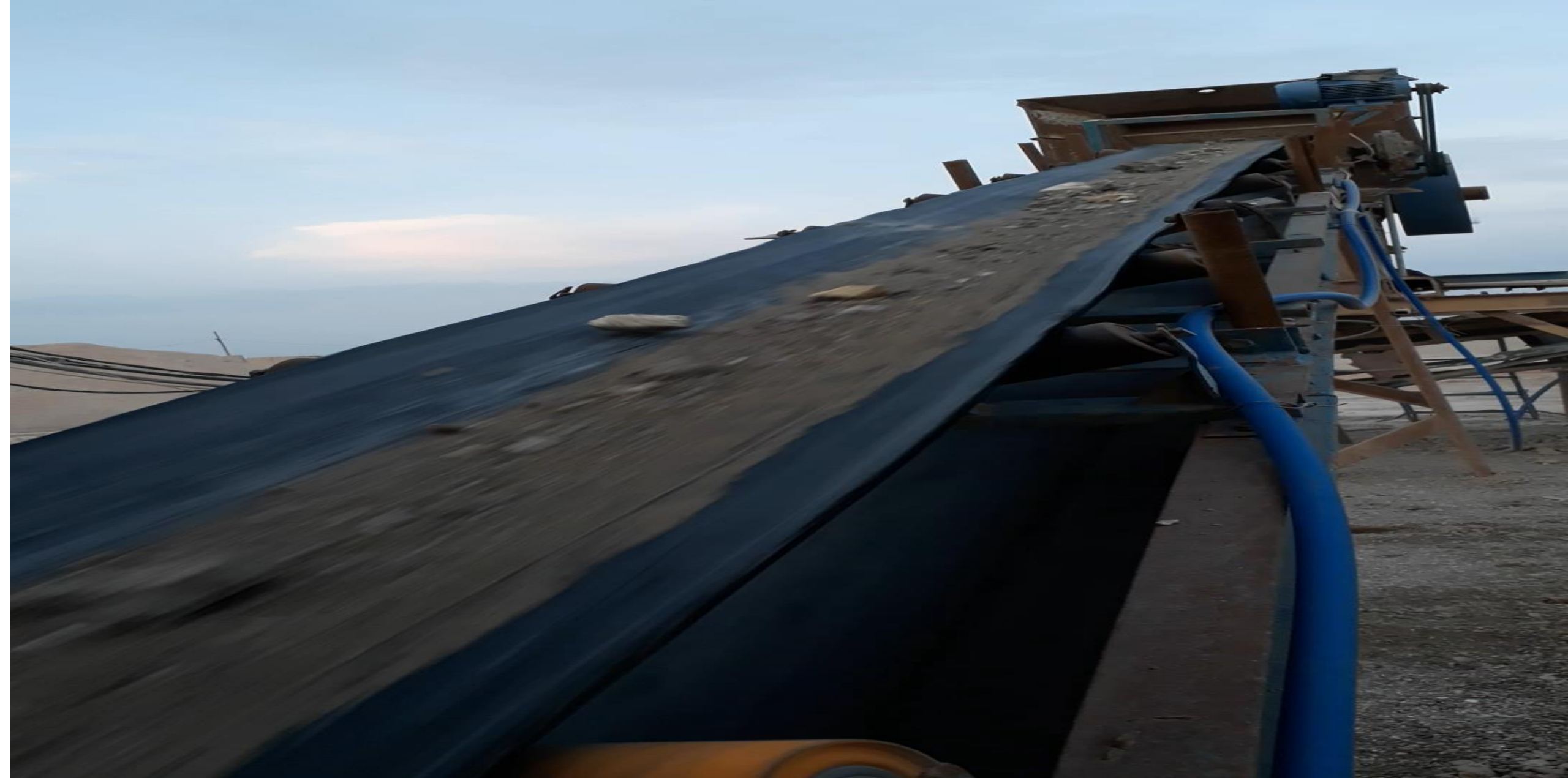
Crushing of debris
