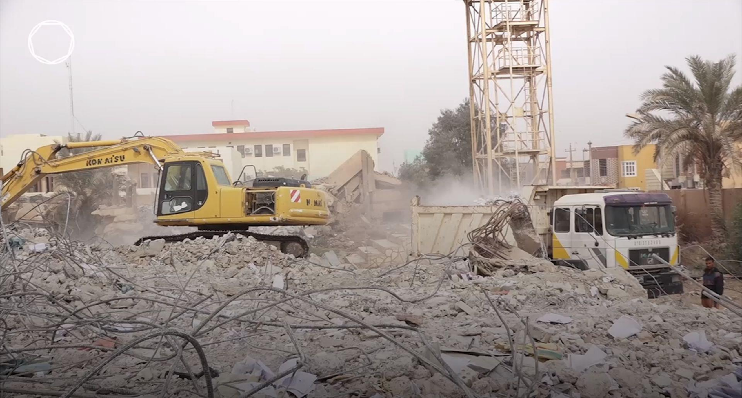
3-Load the trucks with debris to the Al-sarah landfill
