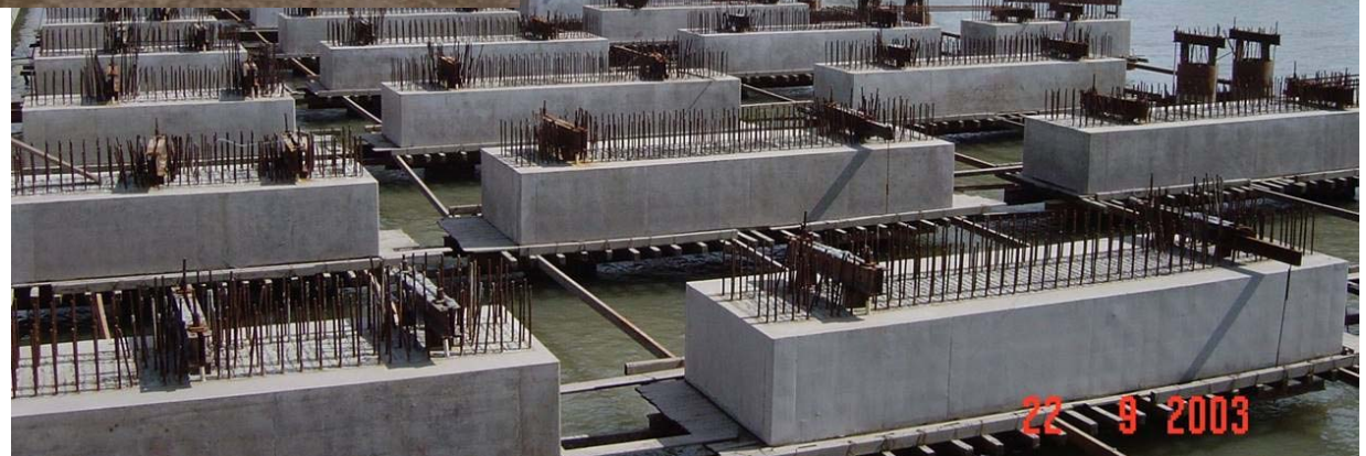
Installation of Concrete Capping Beam
