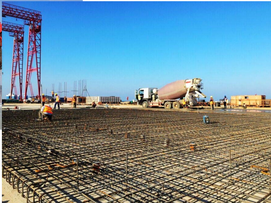
Caisson Precast Yard
