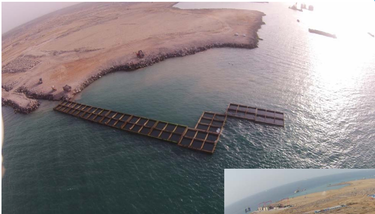
Aerial View of Caisson Installations
