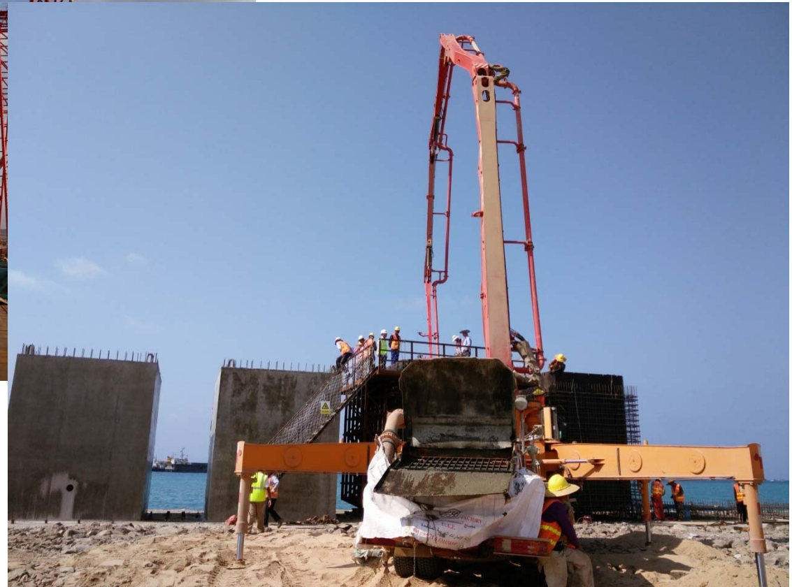
Cast in-situ Concrete
