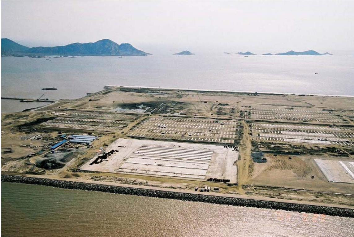
Construction of Container Yard
