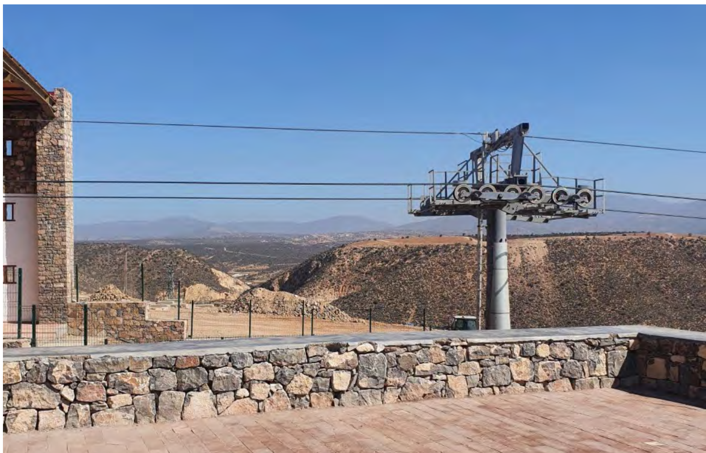
Figure 17. The cable car infrastructure on Oufella hill". The source: UN-Habitat (2022).
