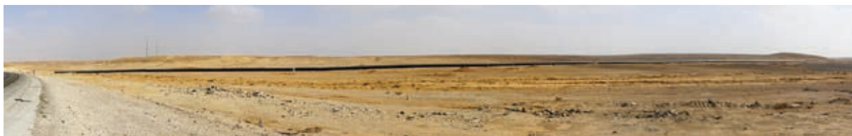
The Disi Water Conveyor, Jordan, 2012. Source: Eileen Maternowski.
