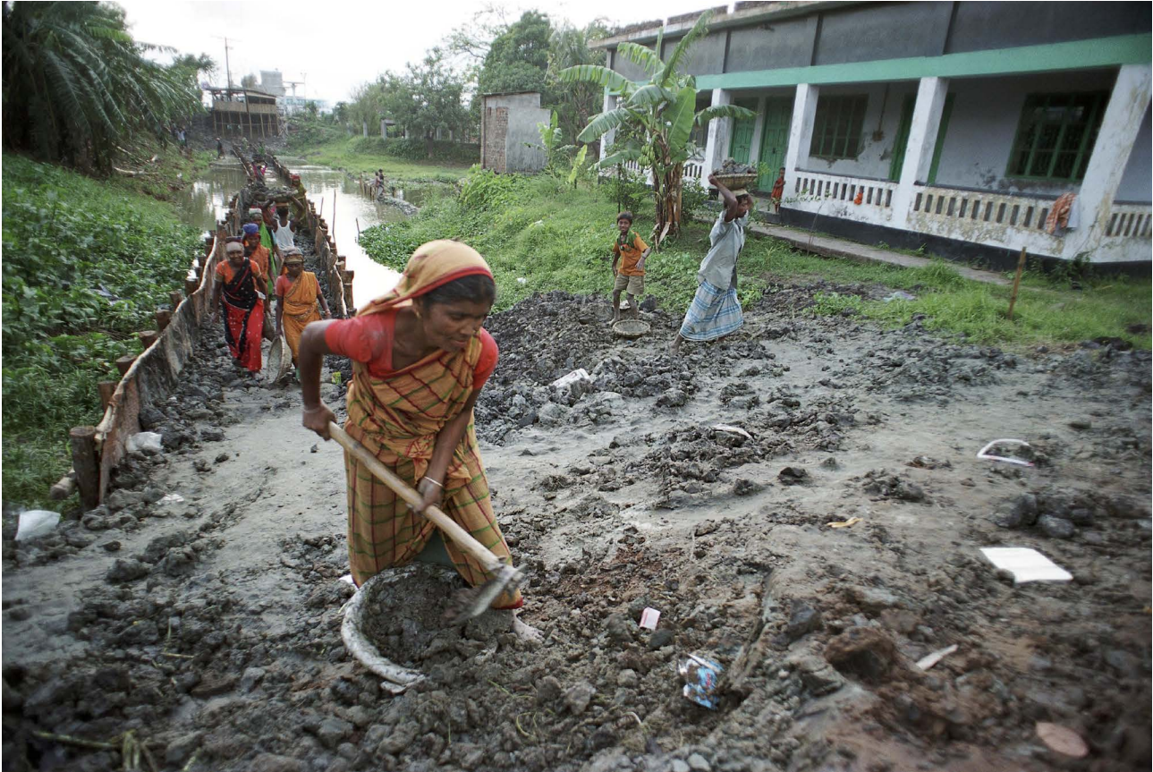
Bangladesh, preparing to build a road. Photo credit: Scott Wallace/World Bank via Flickr, CC BY-NC-ND 2.0
