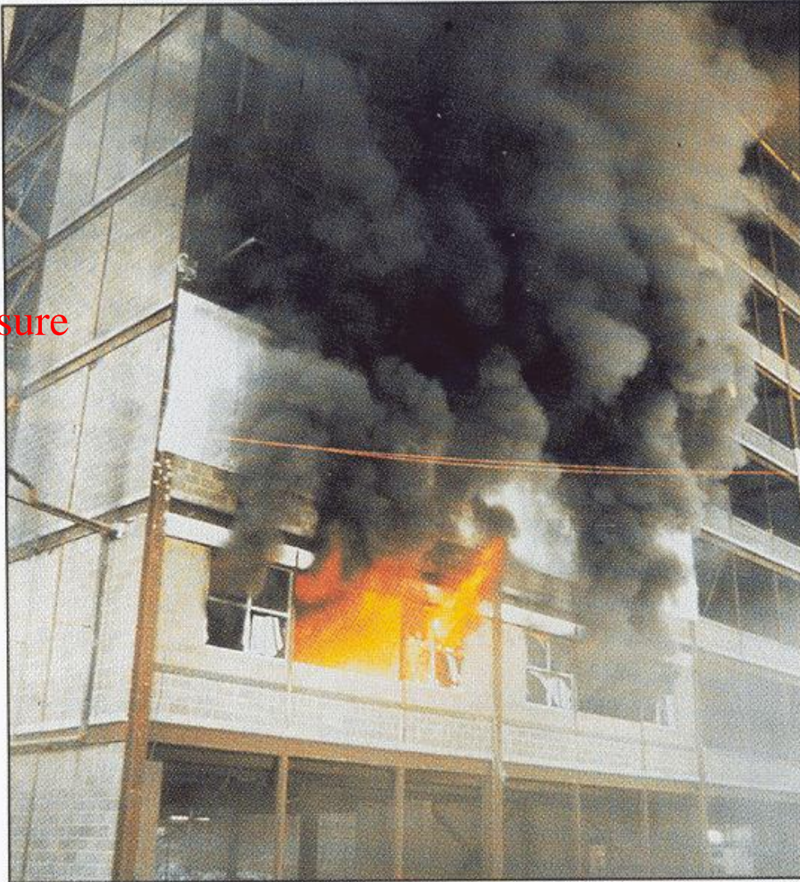
Figure B.3.17 External view of fire
