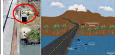
Non-Contact Measurement of Stage & Discharge
