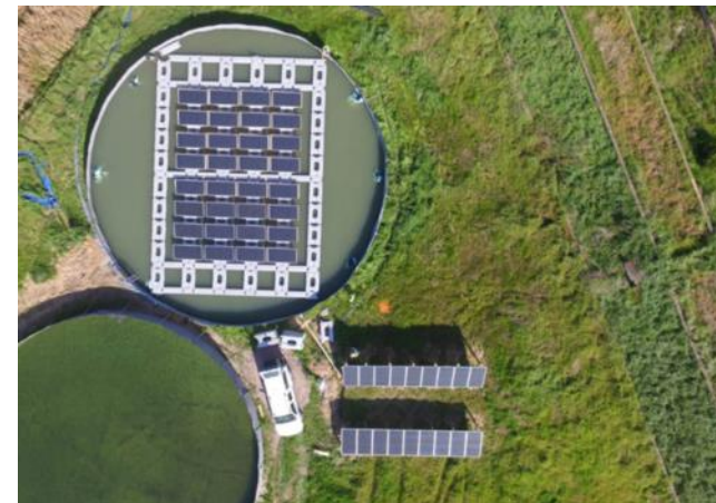
Solar panels in WWTP Lianyungang, China
