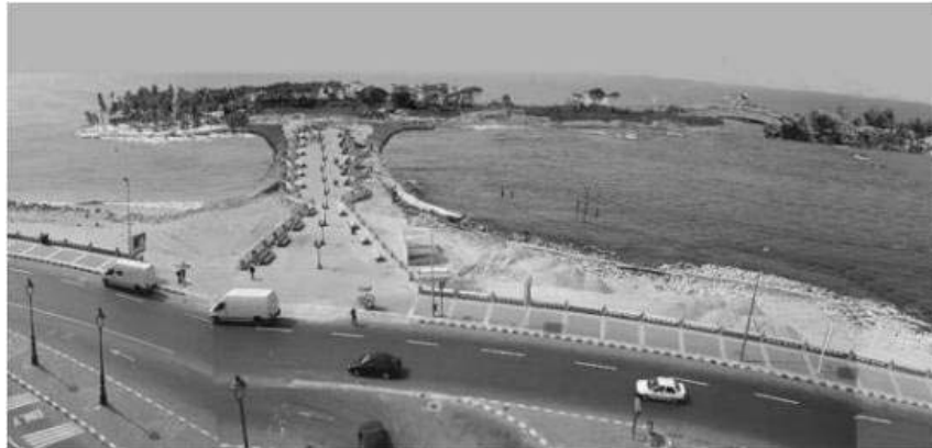
Developing a touristic area and reducing currents and possibly future risks due to sea water rise off shore of Alexandria, Egypt (Al-Raey, 2009)
