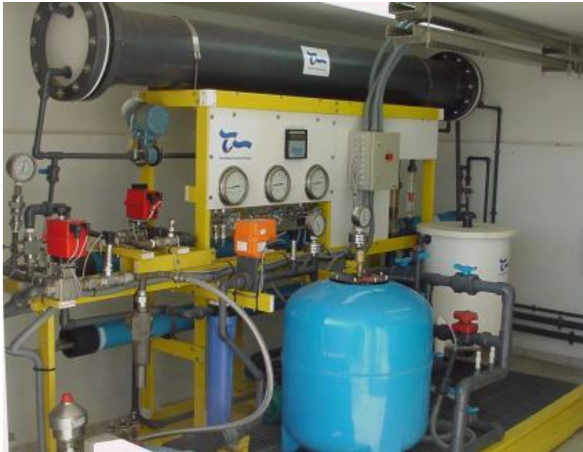
RO unit 750 l/h, 8.4 kWh/m 3 .
