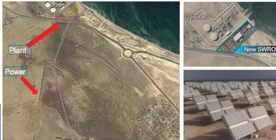
Al-Khafji sewer RO Desalination Using Solar Energy
