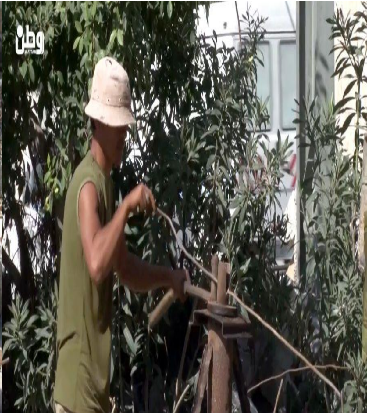
3-Re-adjustment of steel bars
