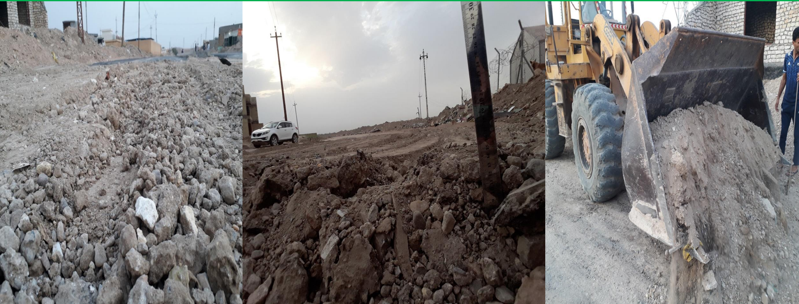
Photo 10, 11.12 shows laying the demolition waste subbase for testing
