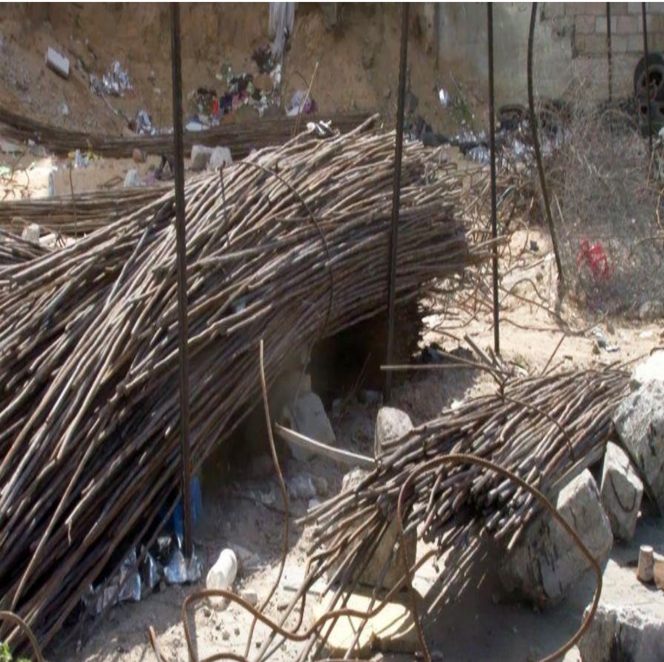
3-Re-adjustment of steel bars
