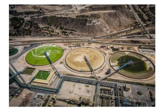
A network of 7 WWTPs to dedicated to provide treated wastewater for reuse in the phosphate enrichment process, and other usages, as an alternative to the freshwater sources. → Benefits: reuse of 15 Mm<sup>3</sup>/Y of urban wastewater
