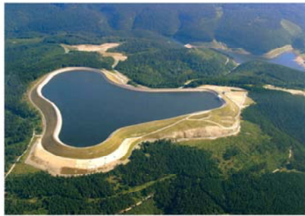
Pumped storage plant in Thuringia (Wirtschaftsspiegel Thüringen, 2011)
