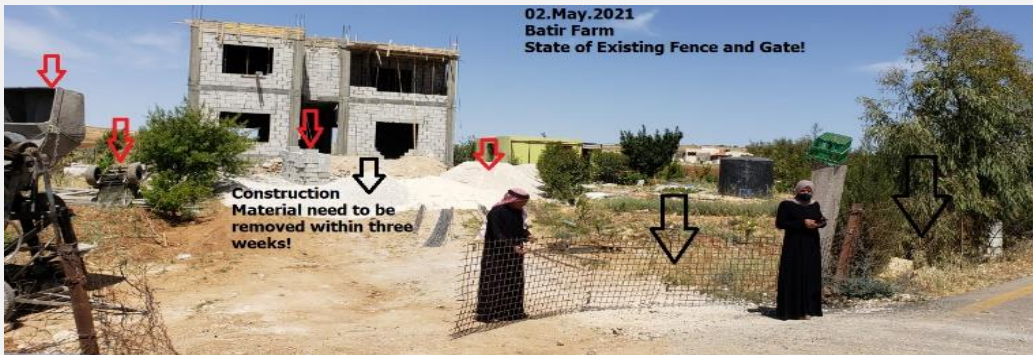
Project #3 (10 kWp): Solar PV off-grid system mounted on an elevated structure for the farm of Mr. Rida Salah in Batir.
