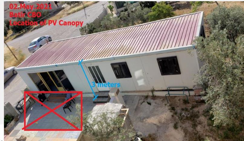
Project #4 (4 kWp): Solar PV on-grid system mounted on an elevated structure for the Shabat Batir Al-Khayriya CBO in Batir.
