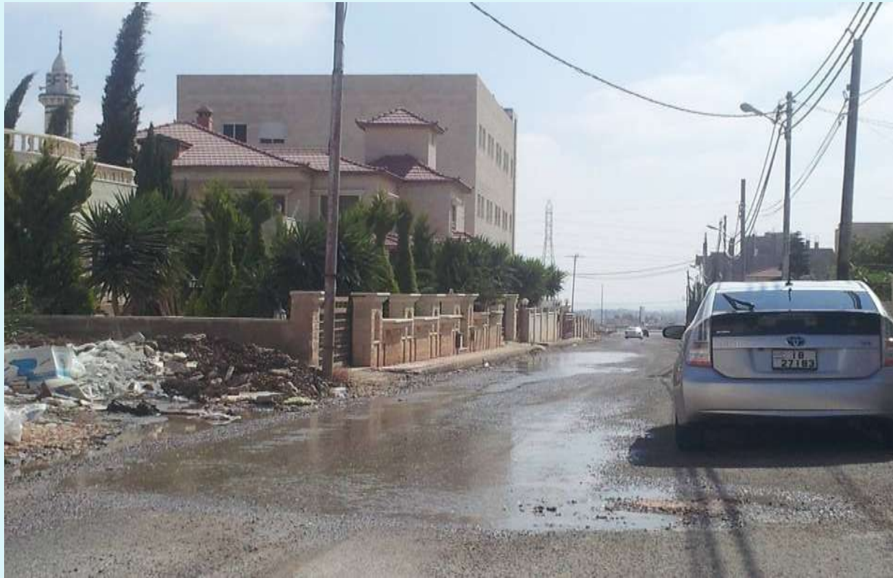
Figure 6 : flooded manhole in a sewage line in Irbid, Jordan, July 2015
